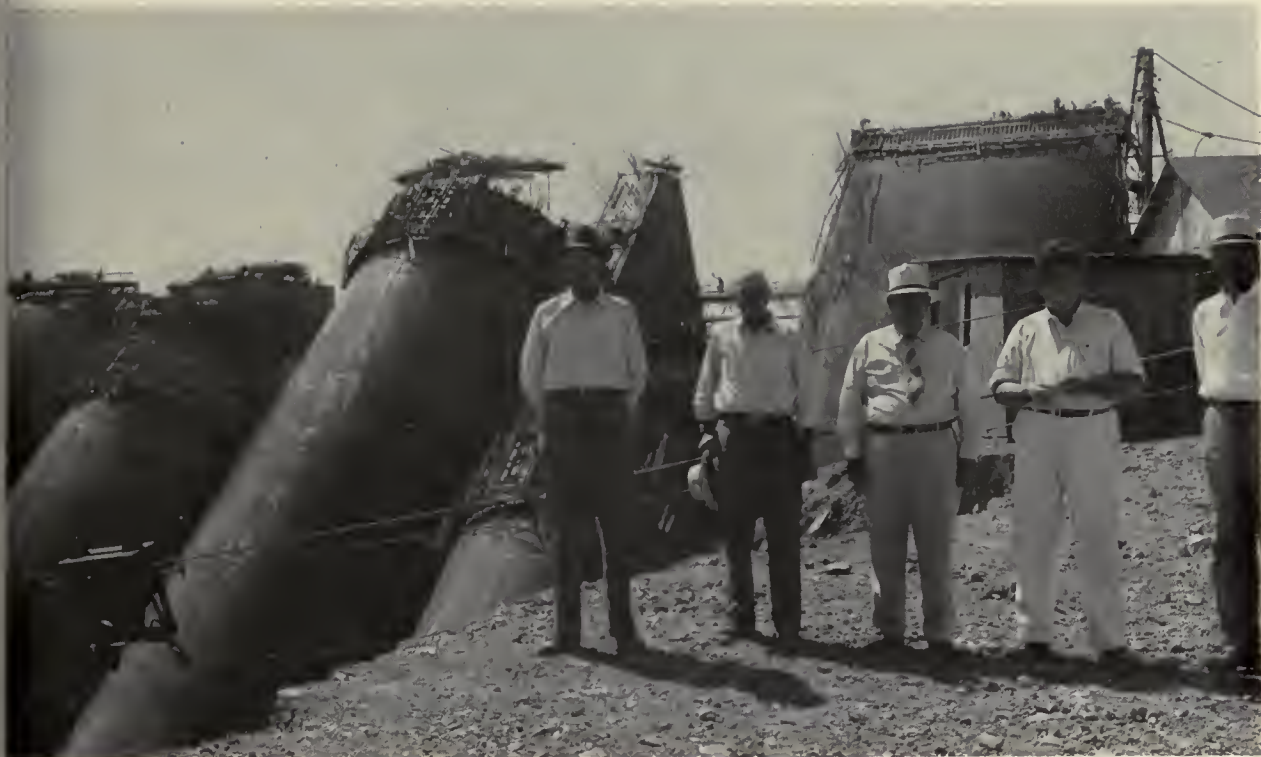
Bartlett Dam on the Verde River near Phoenix, Ariz., shown here under construction, was built during Lin B. Orme's administration as president of the Salt River Valley Water Users' Association.
